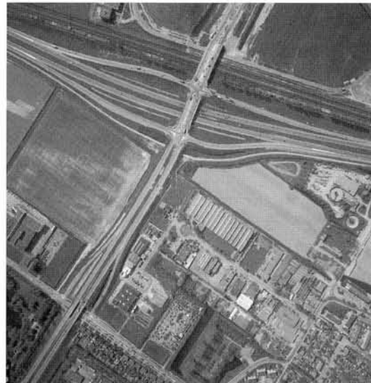
Fig. 5.5 Aerial image of a interchange with Haarlemmermeer solution at the 2-lane motorway A12, part of learning set
