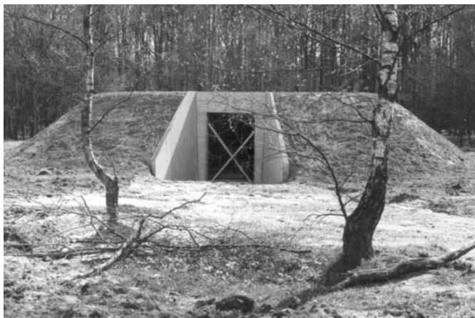
Figure 5: The gravity bunker in Westerbork.
