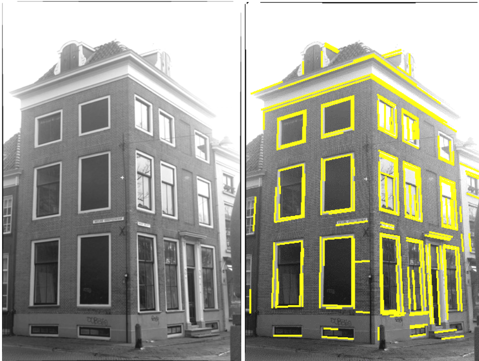
Figure 1: Original image (left). Image overlaid with automatically extracted lines (right). Note the low image contrast on the corner edge where the two façades meet.
